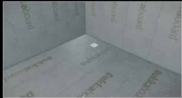
9. Pro Tip - To create a level floor surface meeting the edge of the Dukkaboard Shower-Tray, use the same thickness of Dukkaboard Original-Panel. Continue fitting Dukkaboard Original-Panel to the remainder of the floor, fixing with screws and washers at 300mm centres, starting in the centre of the panels first.
