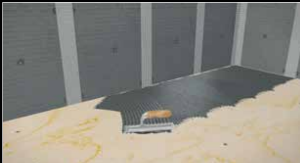
2. Select a trowel with an appropriate notch size for the application.
