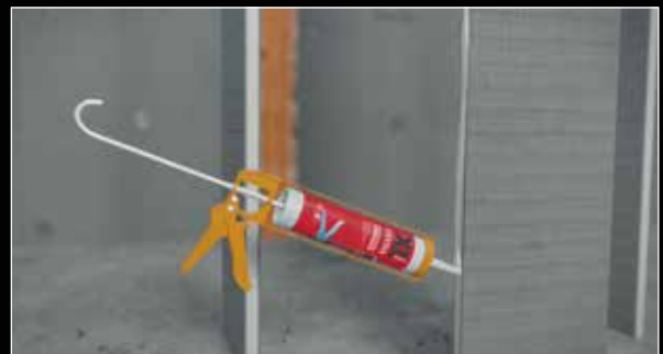
5. Apply glue in a zig-zag pattern for best spread and adhesion. Pro Tip – To accelerate glue curing, moisten contact surfaces before glueing.
