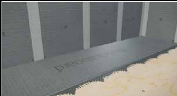
3. When the adhesive is applied, place the Dukkaboard Original-Panels directly onto adhesive layer.
