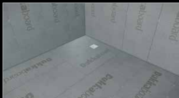
10. Continue fitting Dukkaboard Original-Panel to the remainder of the floor, fixing with screws and washers at 300mm centres, starting in the centre of the panels first.
