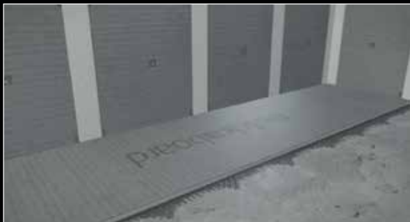
3. When adhesive is applied, place the Dukkaboard Original-Panels directly onto the adhesive layer.
