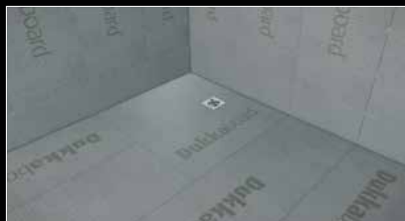
10. Continue fitting Dukkaboard Original-Panels to the remainder of the floor, ensuring all the boards are tamped down and level.
