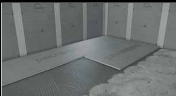
7. Dukkaboard Original-Panels must be laid in brick bond pattern, with staggered joints.
