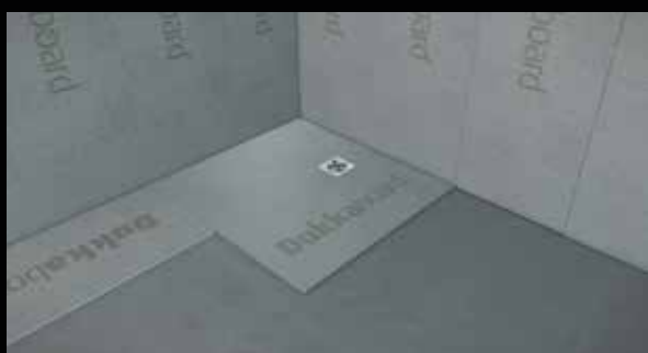
9. Pro Tip - To create a level floor surface meeting the edge of the Dukkaboard Shower-Tray, use the same thickness of Dukkaboard Original-Panel.
