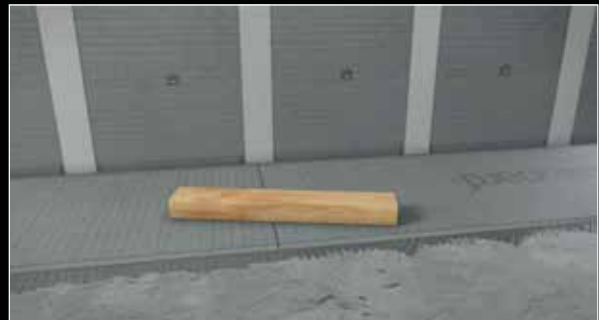
5. Tamp the panel down to ensure that all the panel makes full contact with the adhesive.
