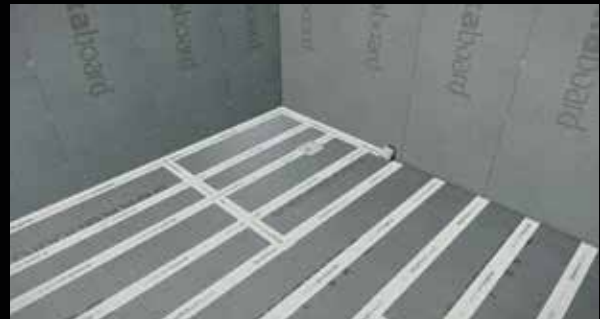
10. Once Dukkaboard Shower-Tray and remaining floor is in place, waterproof all joints with Dukkaboard Waterproof Tape (for wet zones). Ensure all joints and screw heads are taped. If preferred, Dukkaboard Aqua77 Fleece+ and Neo-Flex can be used for all board-to-board joints.
