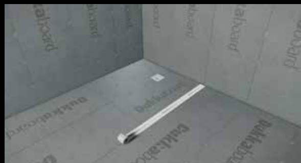
11. Once Dukkaboard Shower-Tray and remaining floor is in place, waterproof all joints with Dukkaboard Waterproof Tape (for wet zones).
