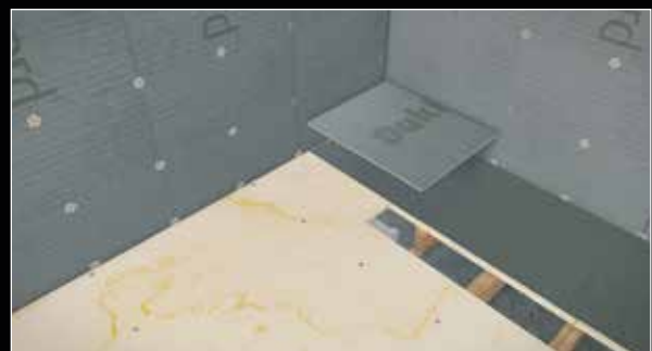
6. Ensure the Dukkaboard Wedge-Panel is correctly rotated so the thicker end backs on to the wall. Place directly onto the adhesive layer.
