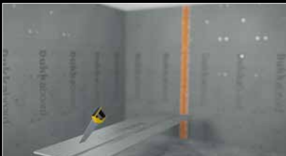
2. Cut pieces of Dukkaboard Original-Panels to create desired size of boxing.
