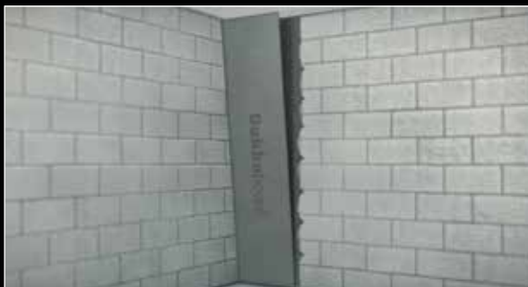
2. Place the Dukkaboard Original-Panel into position.
