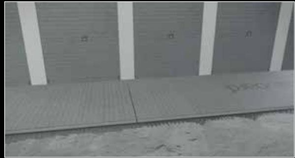
4. Dukkaboard Original-Panels must be firmly butted together.
