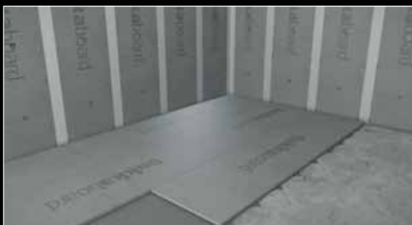
8. For this method, you can use offcuts to help create a brick-bond pattern - however, as a guide, do not use Dukkaboard offcuts smaller than 200x200mm.
