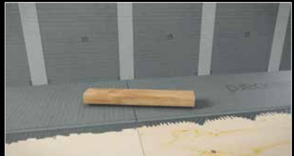
5. Tamp panels down to ensure that all the panel makes full contact with the adhesive.
