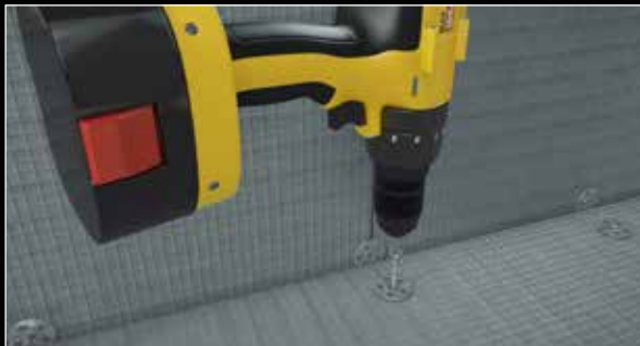
8. Fix the Dukkaboard Shower-Tray in place with screws and washers at 300mm centres, and inset 50mm from edges. Drive screws in firmly to ensure that the washer is flush with board surface. Do not overtighten.
