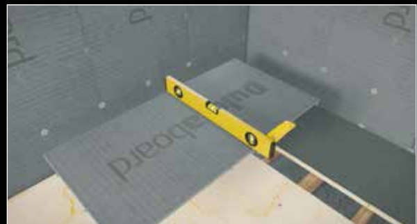
5. Cut to the required size using a Stanley knife and straight edge.
