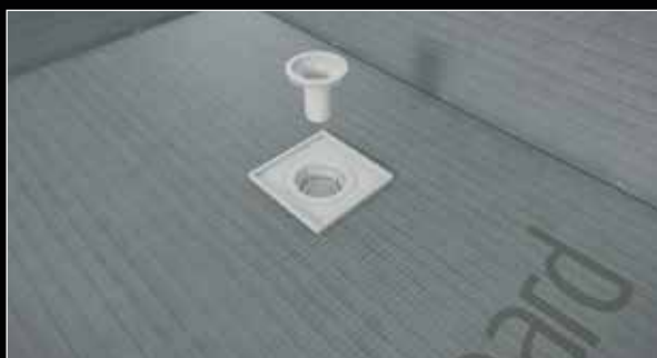
7. Insert bucket and dip tube.
