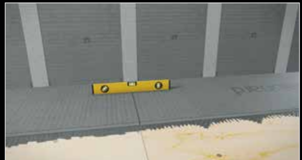
6. Ensure each panel is level with the adjacent panel.
