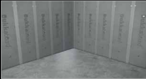
1. Prime the floor using Aqua 77 Pro-Tile Primer before applying adhesive or Dukkaboard.
