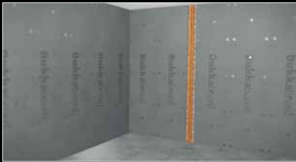
1. Complete surrounding Dukkaboard surfaces before constructing and fitting boxing.
