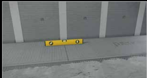
6. Ensure panels are level with the previous panel.
