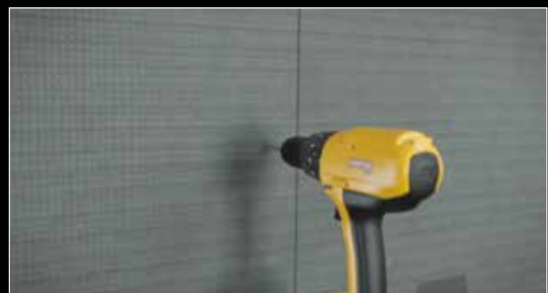
6. Pro Tip - Drill holes for fixing dowels using an 8mm masonry bit.
