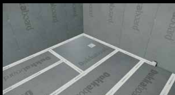
12. Waterproof all joints with Dukkaboard Waterproof Tape (for wet zones). Ensure all joints and screw heads are taped. If preferred, Dukkaboard Aqua77 Fleece+ and Neo-Flex can be used for all board-to-board joints.
