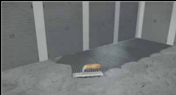
2. Pro Tip - The correct notch size for combing out the adhesive bed is at least double the maximum undulation of the floor, measured under a 1m straight edge.
