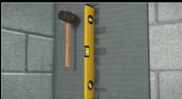
3. Tamp gently to ensure the panel is plumb and is making good contact with adhesive.
