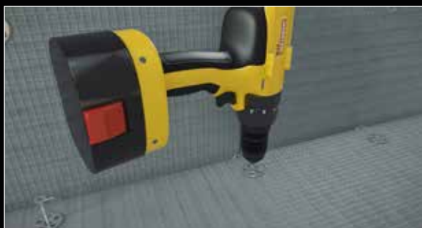
8. Fix Dukkaboard Shower-Tray in place with screws and washers at 300mm centres, and inset 50mm from edges. Drive screws in firmly to ensure that the washer is flush with board surface. Do not overtighten.
