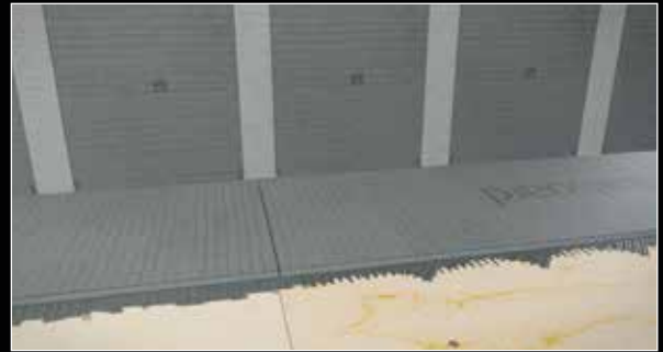
4. Dukkaboard Original-Panels must be firmly butted together.
