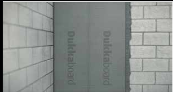
4. Continue application of adhesive and fitting of panels, ensuring all edges are tightly abutted.
