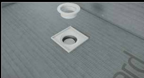
7. Insert the threaded collar to join the Dukkaboard Shower-Tray to the trap.
