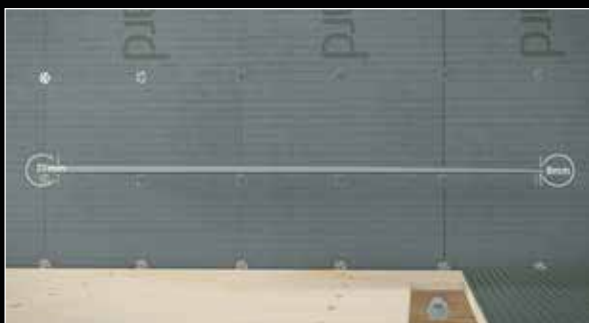
3. The Dukkaboard Wedge-Panel has a gradual gradient to allow for drainage of water. Ensure you always align the lower edge to drain edges or areas.
