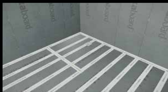
12. Ensure all joints and screw heads are taped. If preferred, Dukkaboard Aqua77 Fleece+ and Neo-Flex can be used for all board-to-board joints.
